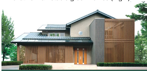
Fig.1. Typical net zero-utility-cost house in Japan (Source: SANYO Homes Co.)
